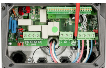
Fig. 23: Connecting the motor cables
